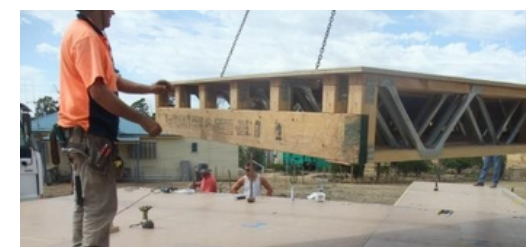
Offsite prefabrication solutions.
