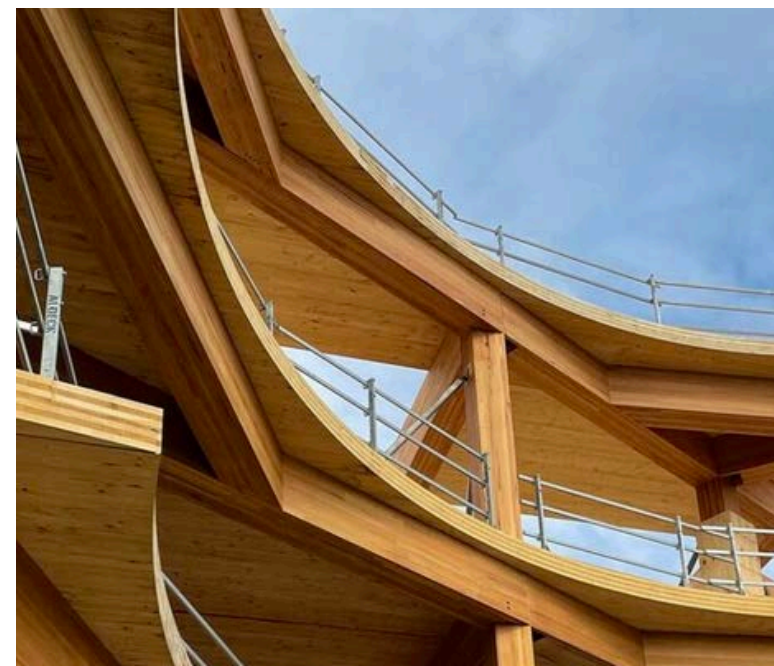
Right: Bendigo Gov Hub - Mass timber (MASSLAM, CLT)
