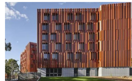
Gilles Hall, Melb Mass timber (CLT) Passive House
