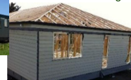
Day 4 & 5- Roof trusses, fascia & gutter
